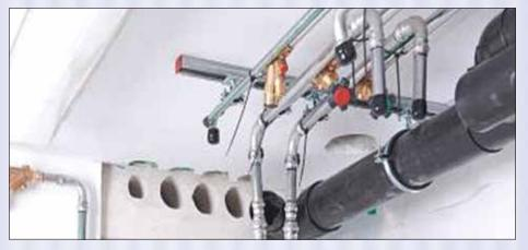
The utmost care was taken in preparing for the assembly in the Antarctic: Openings for the drinking water installation realised with the Viega "Sanpress Inox" system made of stainless steel 1.4521. (Photo: Viega)
